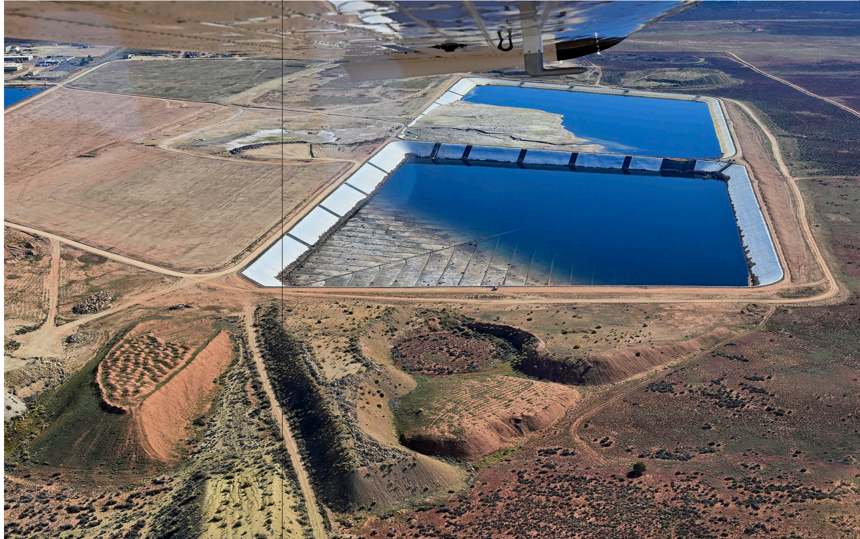
Waste pits known as Cell 4a (top) and Cell 4b (bottom) at the White Mesa Mill. By law, solid materials in the holding and processing ponds at the mill are required to be covered in liquid, which acts as a barrier to cancer-causing radon gas emitted by the materials in the pond. TIM PETERSON, ECOFLIGHT
